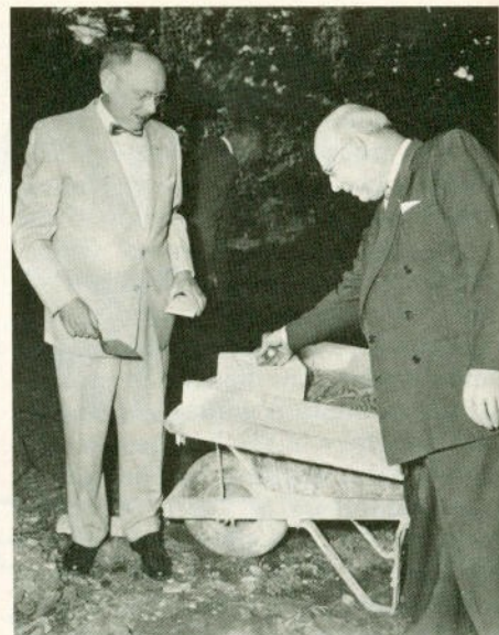
Laying the cornerstone of the "new" Central Office in Oxford in 1956 are Grand president J. Harry Feltham (left) and Past Grand President John L. McKewen.
