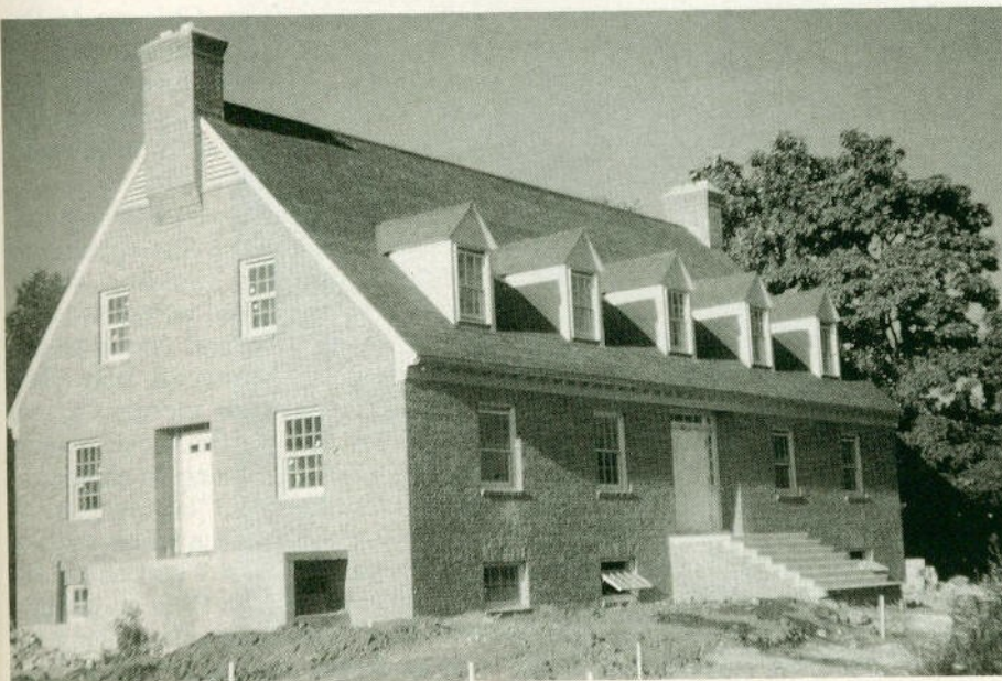
As the summer of 1956 came to an end, the construction of The Central Office progressed toward a September 1 occupancy date.
