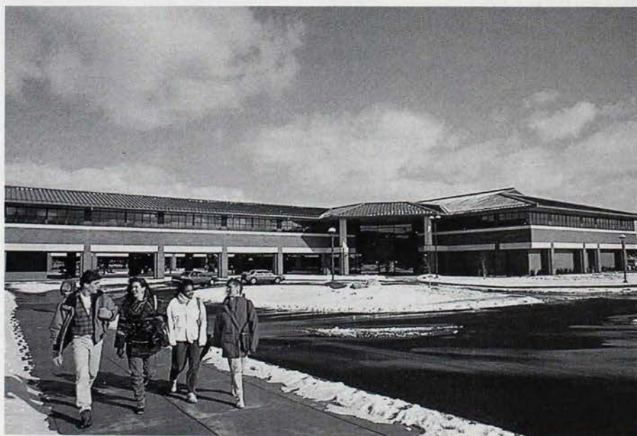
The new home of the Haworth College of Business at Western Michigan University. (Photo courtesy of Western Michigan University)
