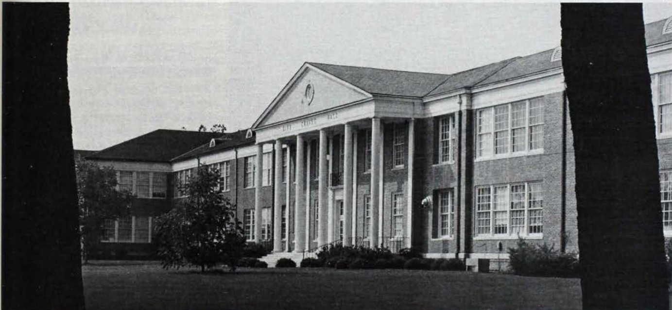
Bibb Graves Hall is only one example of the Georgian-style architecture on the campus of Livingston University, home of Lambda Rho Chapter.
