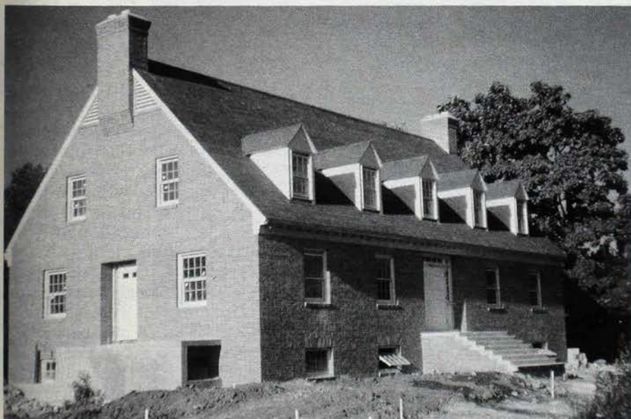
As the summer of 1956 came to an end, the construction of The Central Office progressed toward a September 1 occupancy date.
