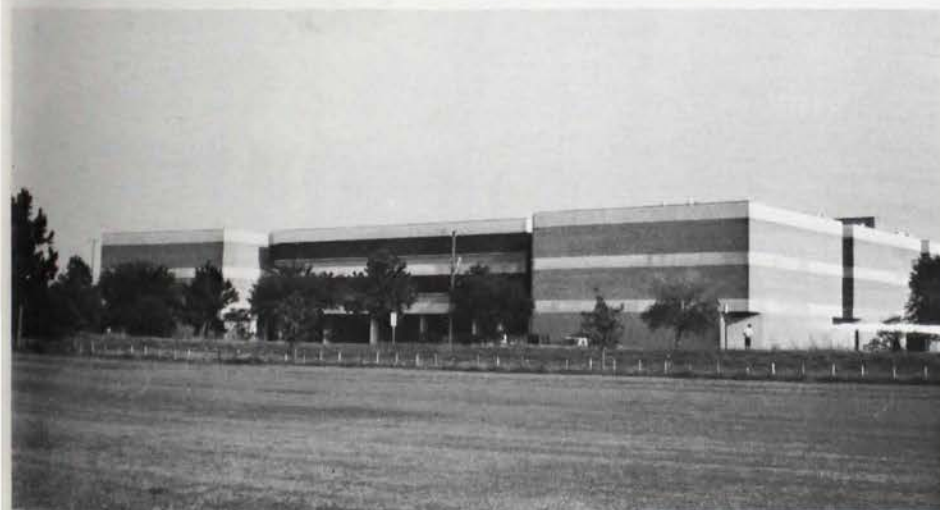
The new $16.5 million Center for Engineering and Business Administration at Louisiana State, home for Beta Zeta Chapter.
