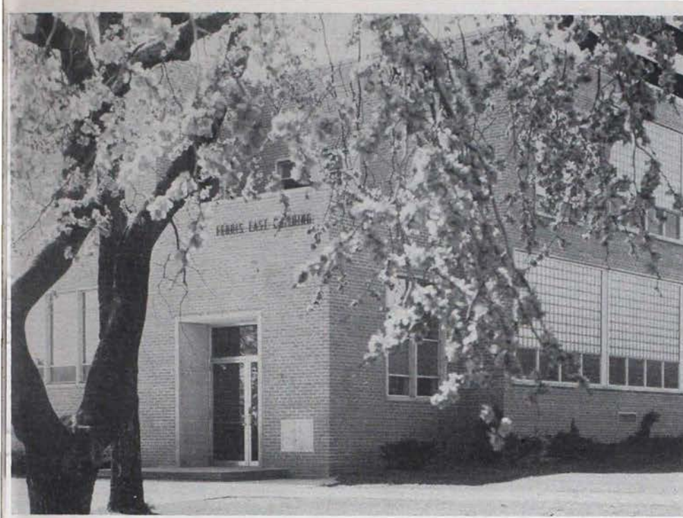
FERRIS EAST BUILDING contains the Division of Commerce at Ferris Institute.
