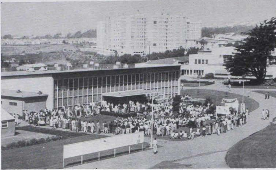
STUDENTS OF SAN FRANCISCO STATE COLLEGE gather in front of the campus cafeteria for a lawn concert. To the right is the College Gym and in the background is the modern Stonestown Apartments.
