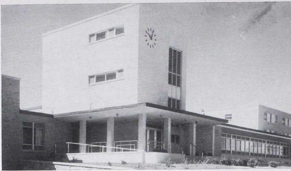
ANOTHER NEW and attractive building on the Ferris Institute Campus is Masselink Commons which serves as a dormitory.
