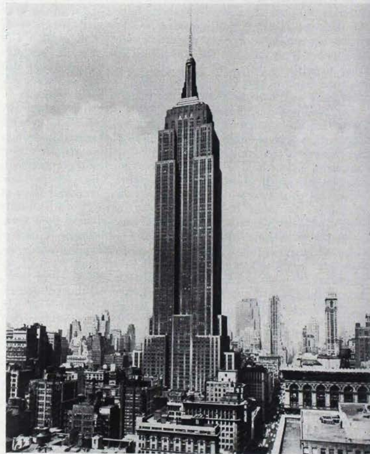
THE EMPIRE STATE BUILDING in New York City is the tallest building in the world with 102 stories. Deltasigs attending the 21st Grand Chapter Congress this summer will have an opportunity to visit the observatory on its uppermost floor.
