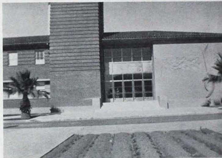
THIS BEAUTIFUL BUILDING is the new Student Union at the University of Arizona. The installation ceremonies and banquet of Gamma Psi Chapter were held here in November just prior to its completion.
